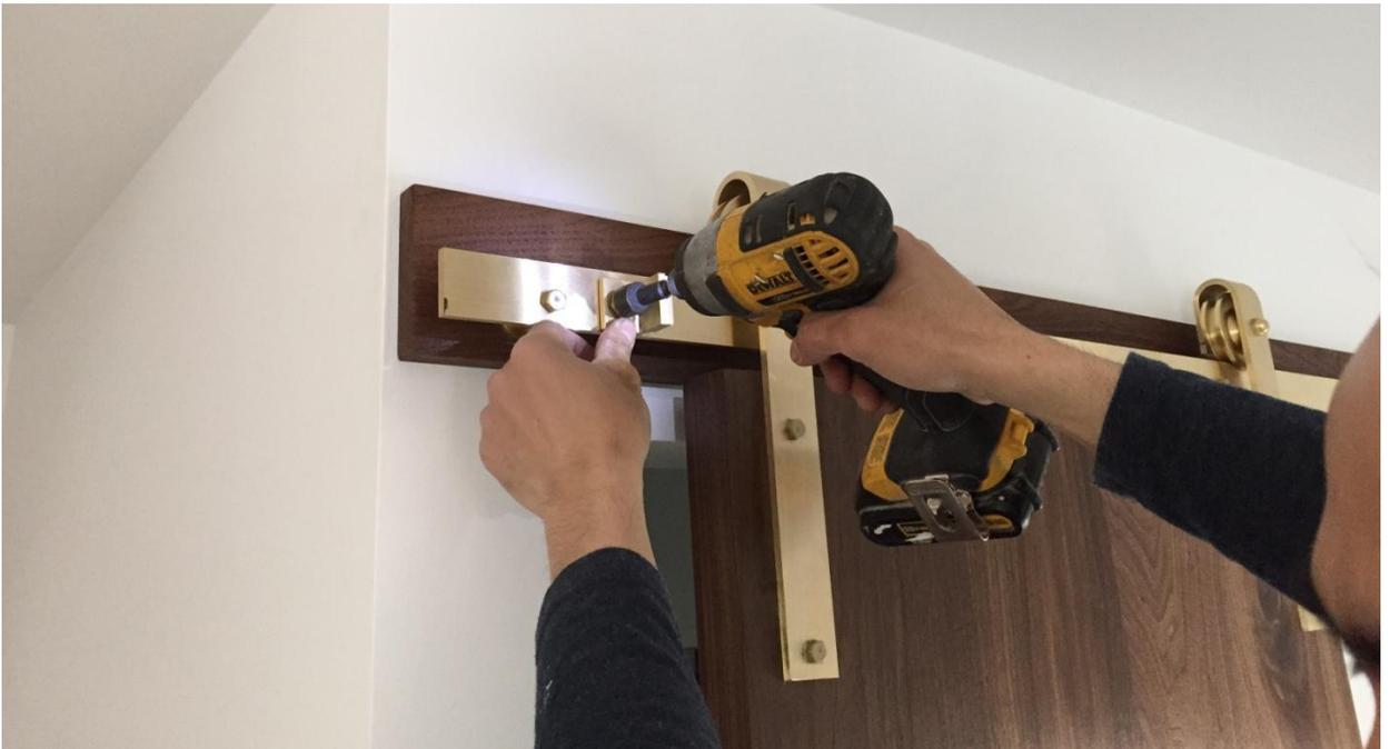
NOTE: Usually, stoppers can be installed on the last hole on both ends of the track so that new holes do not need to be drilled
