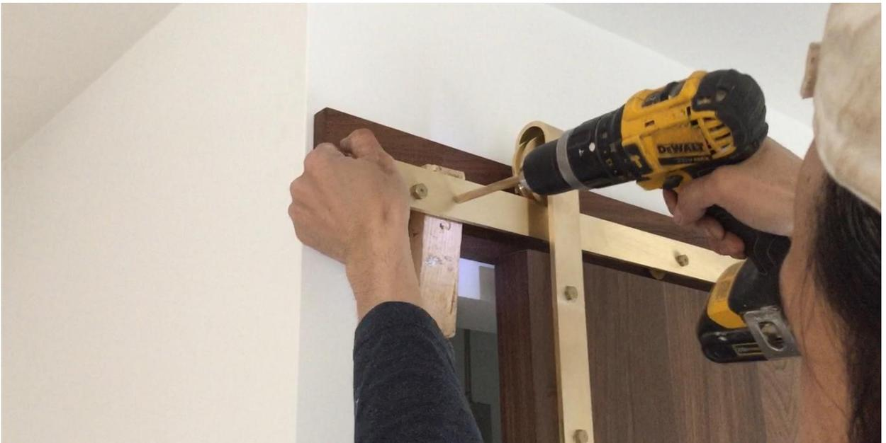
Use provided nuts and bolts to fasten the stoppers to the track.
