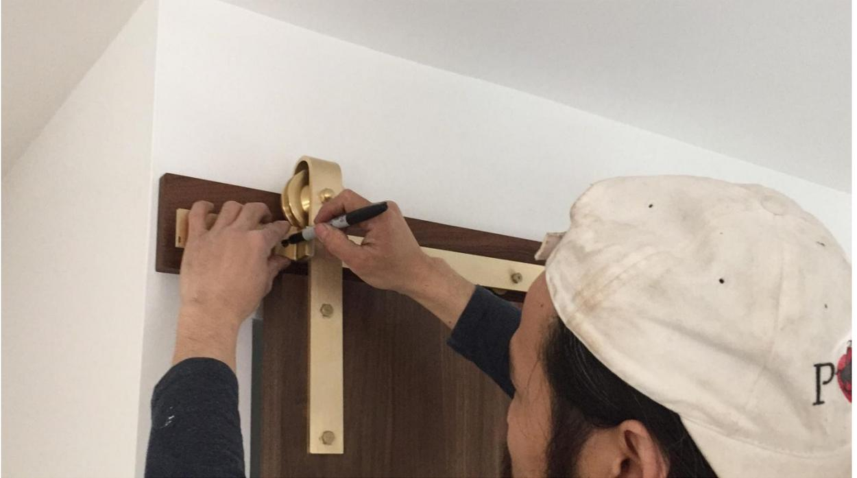
Use 5/16" drill bit to drill holes for stopper. It is a good idea to put a piece of wood behind the track directly behind the hole being drill to prevent drilling into the wood block
