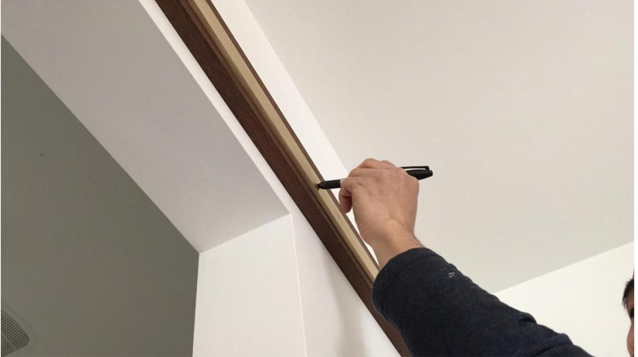
Remove the track, then use 3/16" drill bit to drill marked holes
