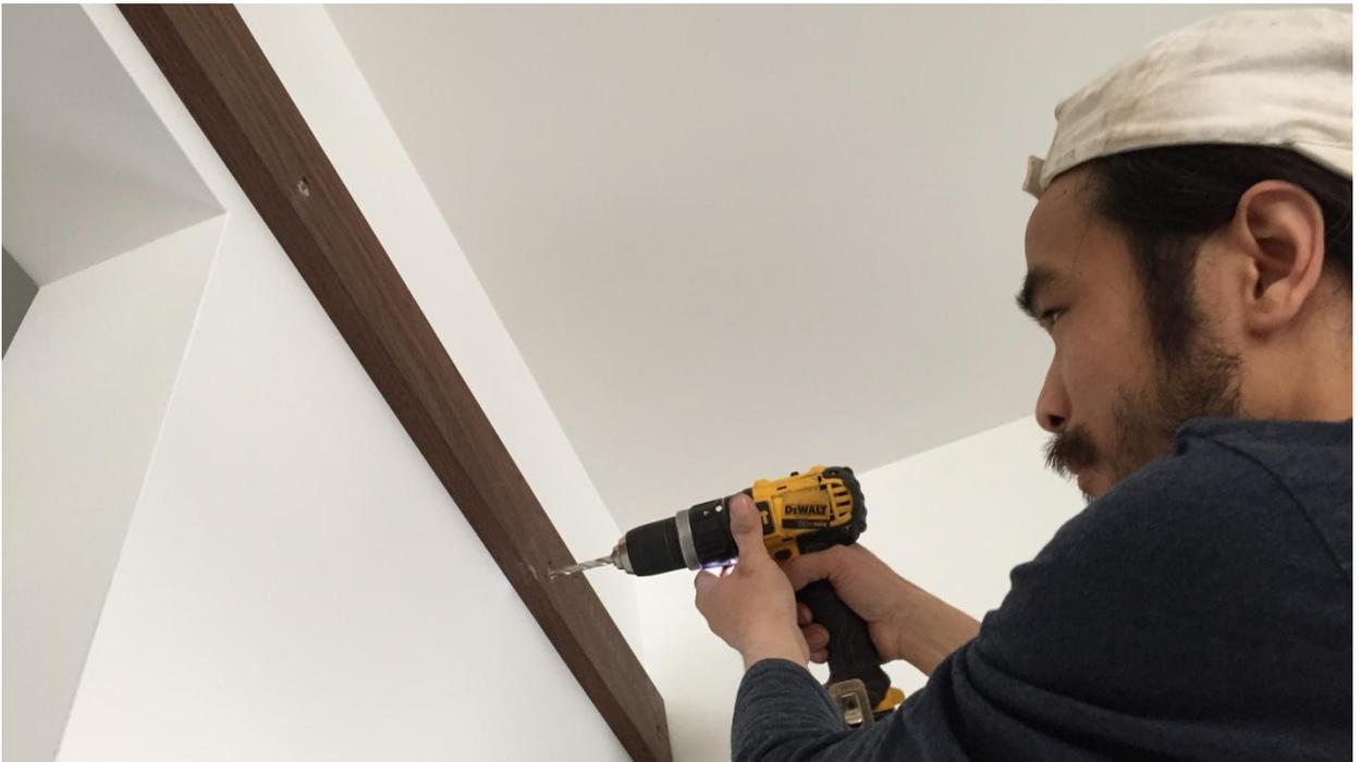
Use provided 5/16" x 4" lag bolts and spacers to fasten the track to the wood block. Note, the flanges on the spacers are to face the wood block. Check for level and adjust if necessary.
