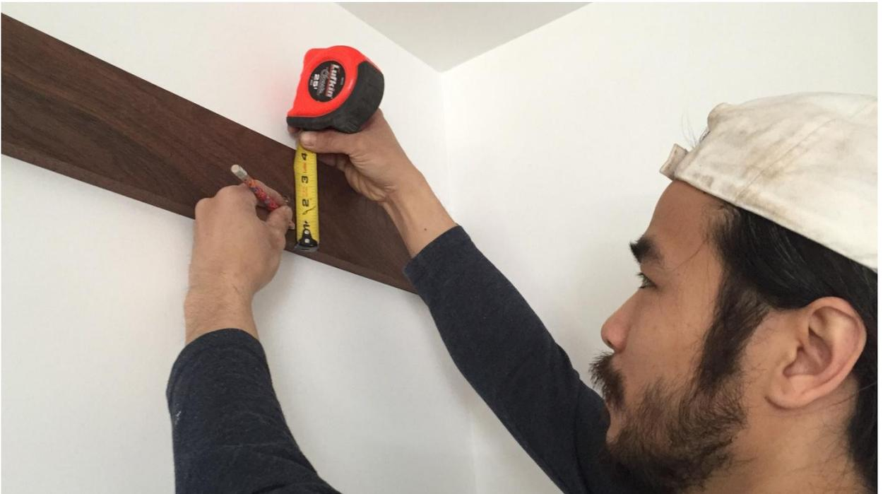
Lay the track on the wood block and mark the drilled holes onto the wood block. Make sure the track is leveled.
