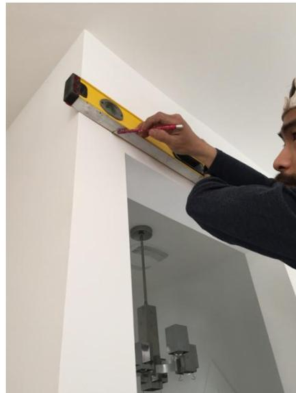
Use 3" long size 8 construction screws (not provided) to fasten the wood block to the wall studs. 2 screws are recommended for every stud. Test for level.
