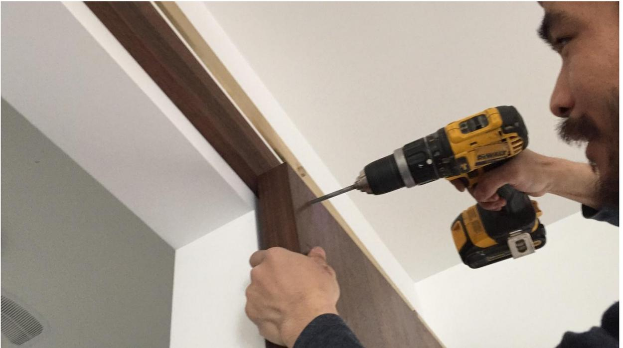
Use provided 5/16" x 1.5" lag bolts to fasten the hangers on the door.
